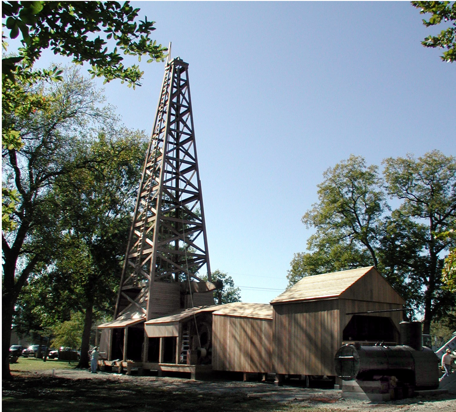
The rig nears completion and prepared for operation.
