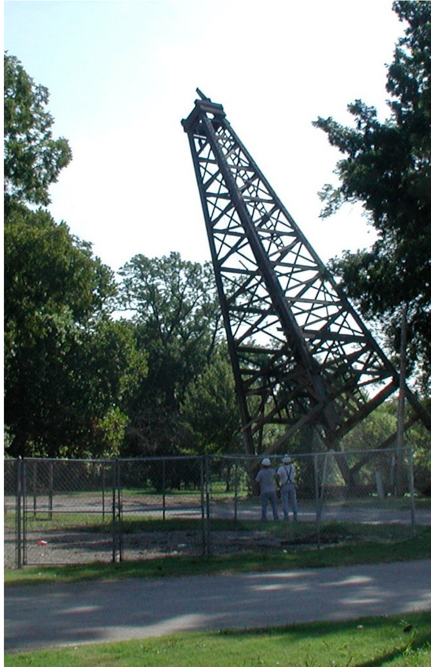
The second derrick reproduction, badly deteriorated, is toppled on Aug. 15, 2007.
