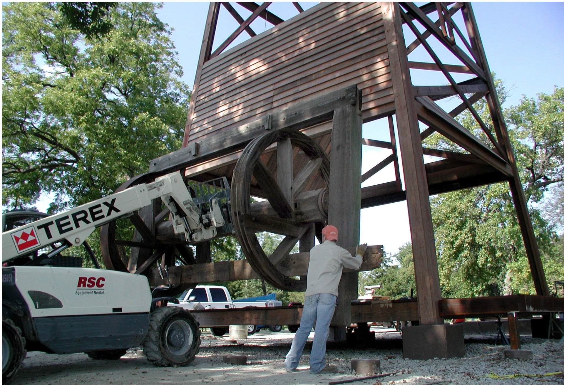
The “bull wheel” cable spool that was salvaged from previous rig reproduction and installed in the new derrick.
