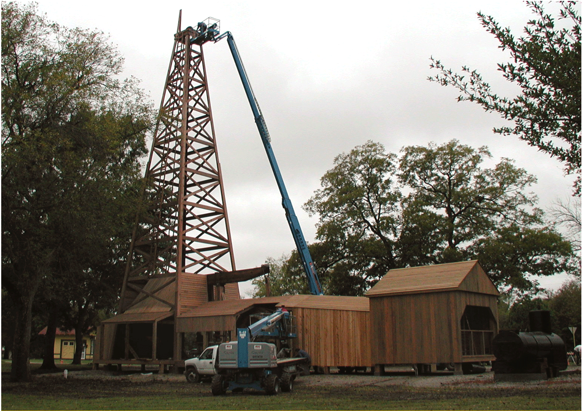
The derrick is “topped off” with the installation of a large pulley in the rig crown.
